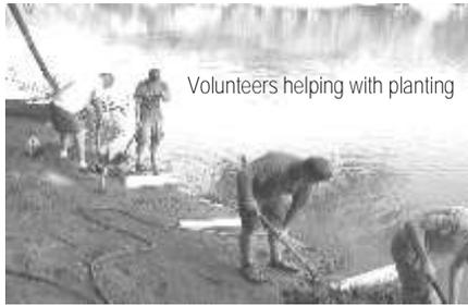
low branches. The hole is sealed and the branches eventually leaf out and produce roots to stabilize the soil. The depth of planting ensures the willow shoots aren't washed out before they become firmly rooted in place.
